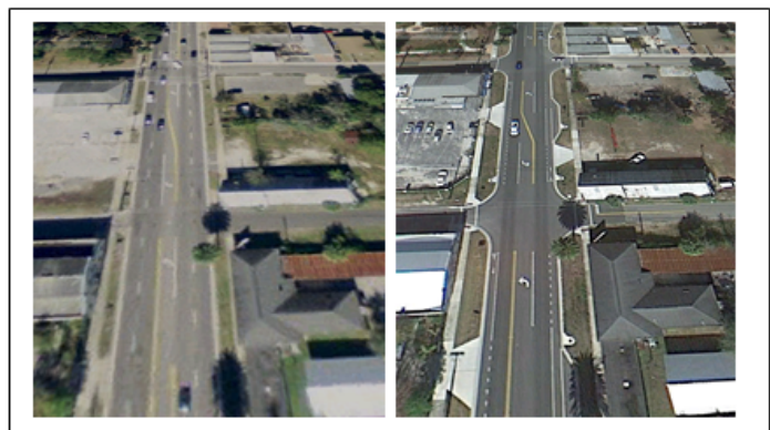
Figure 2: Main Street Corridor - Before and After
